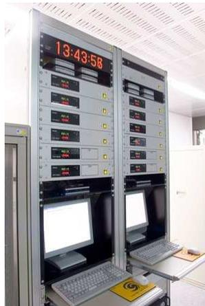
**Figure 4. Telephone JJY System.**
